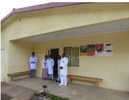
The pre-existing health post after renovation.
