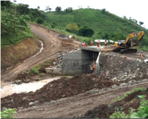
Roads and culverts built for the community.
