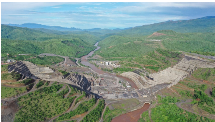
The construction project currently in progress.
