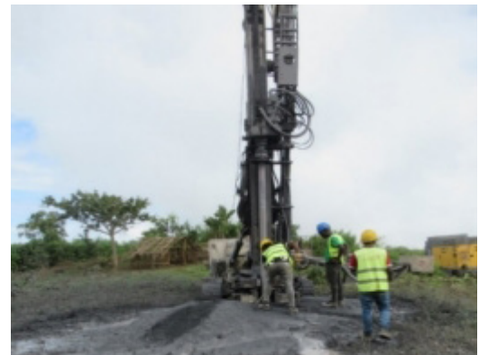
Drilling of water wells.
