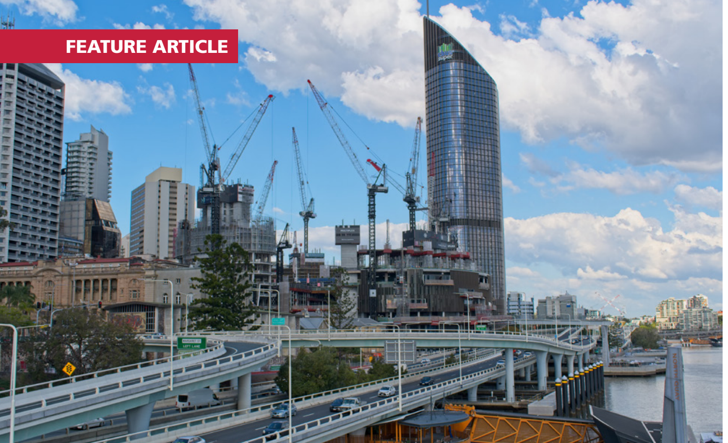
Construction activity near Riverside Expressway, Brisbane, Australia. Credit: Shutterstock/my_ photos
