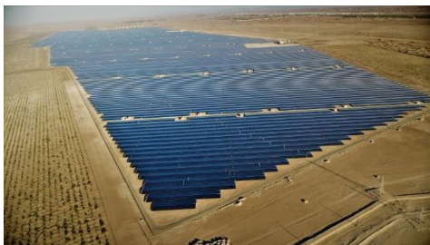
The Sweihan power project Power Division
