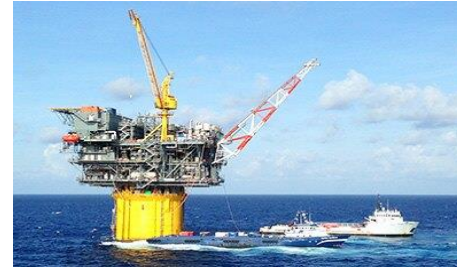
Gulfstar One, LLC Energy Infrastructure
