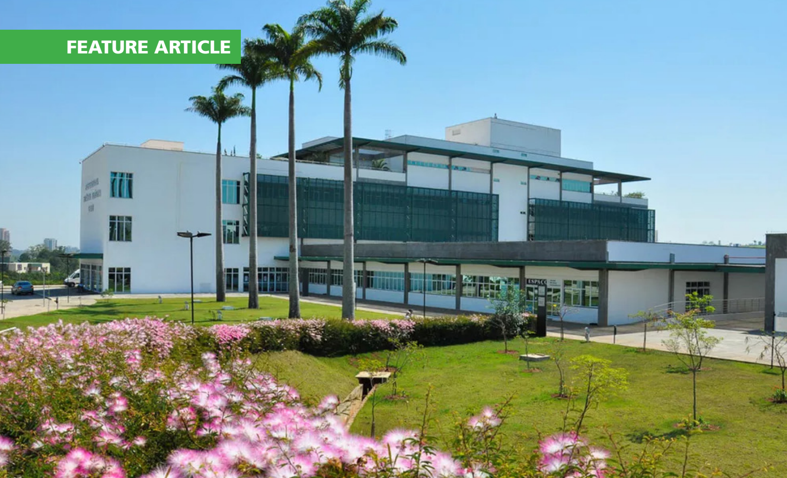
Municipality of Itu Headquarters Building. Credit: Prefeitura de Itu/Divulgação
